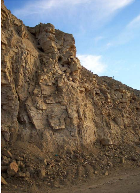
Fig. 4.7 Loose final faces resulting from production blasting
