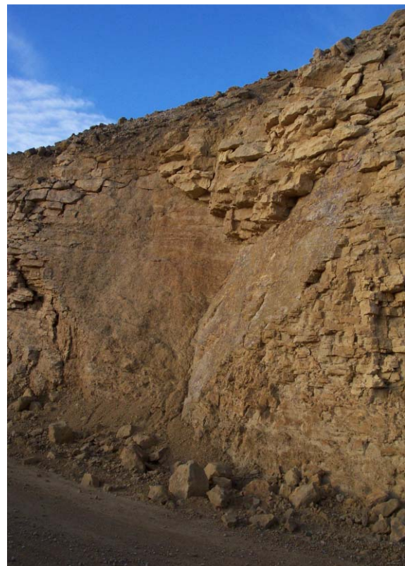
Fig. 5.7 Wedge failure in a magnesian limestone quarry (note continuing unravelling of upper slope)
