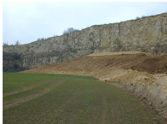
Fig. 6.41 Partial tipping against face (incorporating a rockfall protection bund in front of the rock face)
