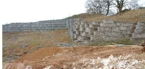
Fig. 6.11 Man-made support buttressing with gabions
