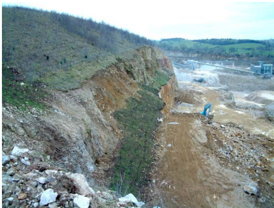
Fig. 6.42 Tip above a final slope with no rock head bench and lower bench filled with forward sloping waste
