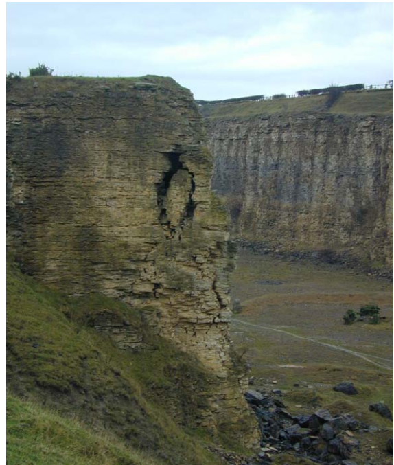
Fig. 5.9 Columnar collapse and rockfall in nose left in face in a magnesien limestone quarry
