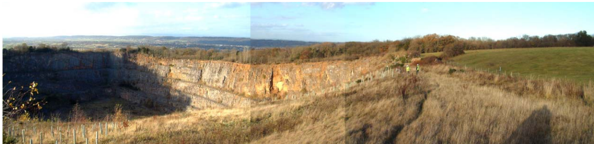
Fig. 6.26 Tipping from floor to rim over a blasted bench system
