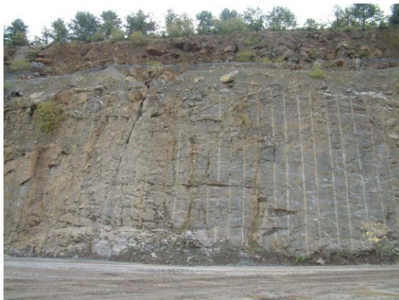
Fig. 6.35 Pre-split blast holes in a final rock face (Note upper edge protection is not secure)
