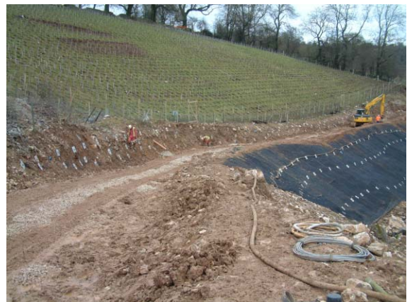
Fig. 6.36 Matting pegged to a rubble slope to protect lower slopes from rockfall
