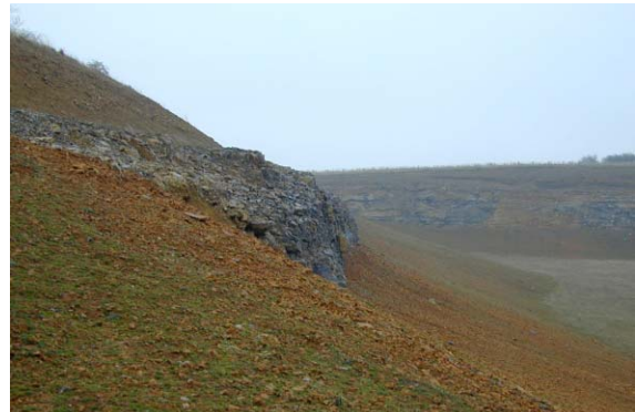
Fig. 6.29 Rock feature protruding from a long backfill buttress; the feature being a rounded bench crest of Fig. 4.6
