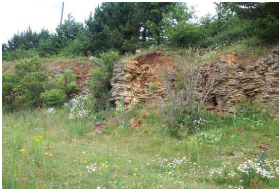
i Unstable final faces produced by face shovel excavation
