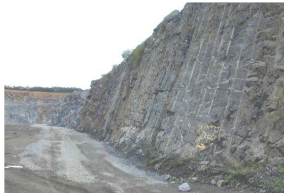
Fig. 4.8 Pre-split faces (near) and production blasted faces (beyond)
