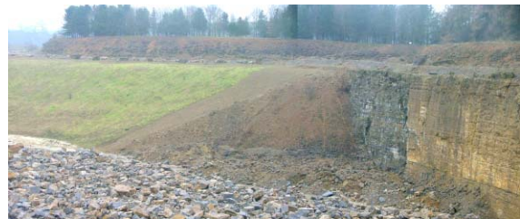
Fig. 6.40 Successful tipping against face
