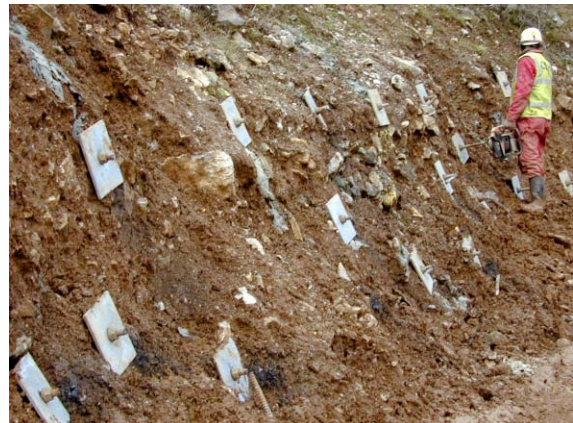
Fig. 6.20 Soil nailing as part of a stabilisation project shown in Fig. 6.21
