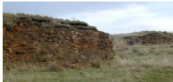
Fig. 6.30 Floor raising by backfill to support the lower section of a final slope
