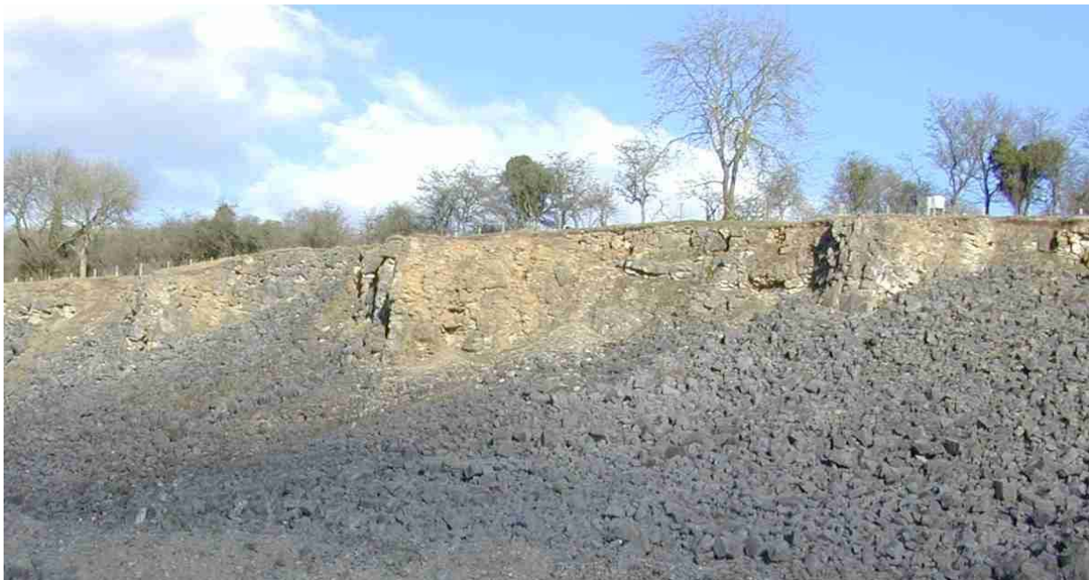
Fig. 4.4 Headwall buttresses and scree slope formed by blasting. Note damage to buttresses
