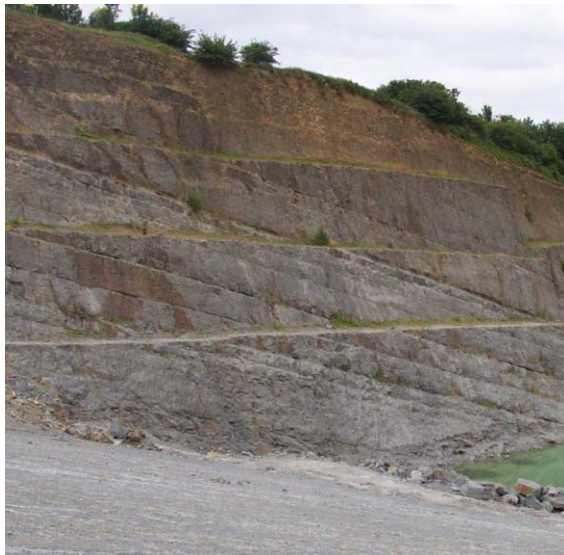
Fig. 8.1 Clean, final, low bench height slope faces excavated by breaker in an SSSI (Note access provided by benches to inclined strata)
