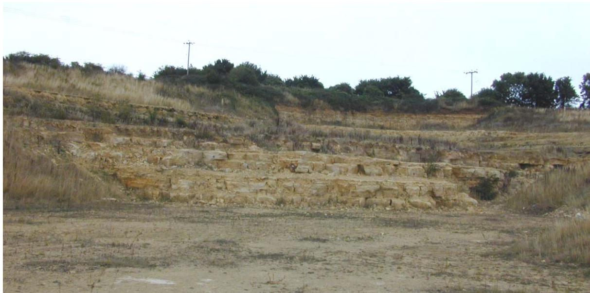
Fig. 8.2 Low benching of rock for long term safe access to a geological SSSI
