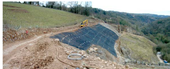
Fig. 6.21 Stabilisation of superficial materials above a steep rock slope to protect land behind the quarry limits
